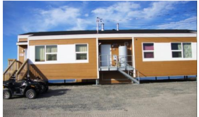
Figure 3. Field monitoring of traditional house in Kuujuaq, Nunavik with attic ventilated through wall cavity behind cladding and filter membranes to prevent infiltration
