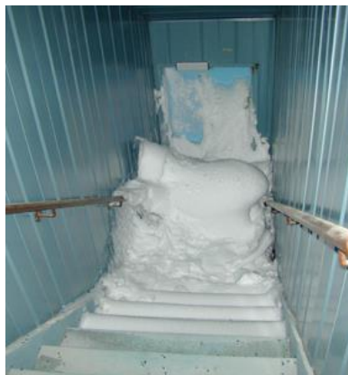
Figure 1. Fine snow ("sugar snow") penetrates any small crevice and accumulates in ventilated attics and doorways in the winter, and melts as temperatures rise.
