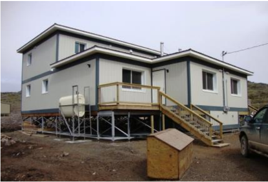
Figure 2. Field monitoring of SIP house with unventilated attic built in Iqaluit in 2012 by Kott with remote real time feedback while occupied
